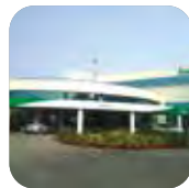
Fortis Escorts Hospital Faridabad
